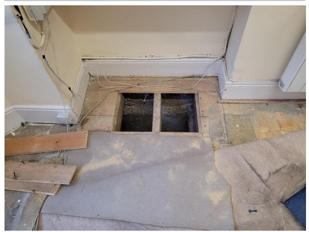
Figure 28. Showing the area opened up in the ground floor sitting room where we exposed the physical DPC.
