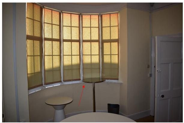
Figure 26. Showing the ground floor dining room. Note the dampness underneath the window sill due to poor detailing.
