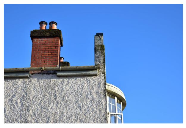
Figure 34. Showing the stained parapet from water running off the coping. This has caused dampness on the ground floor west wall.
