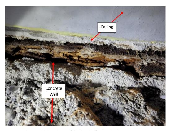
Figure 11. Showing an image of the above sketch where the plaster was removed.
