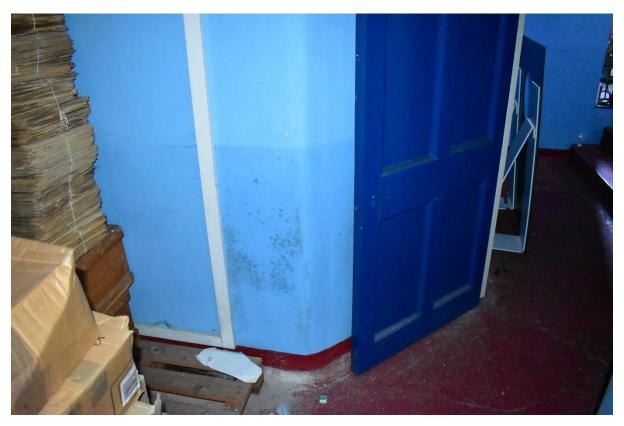
Figure 29. Showing the mould visible at the lower ground floor level.
