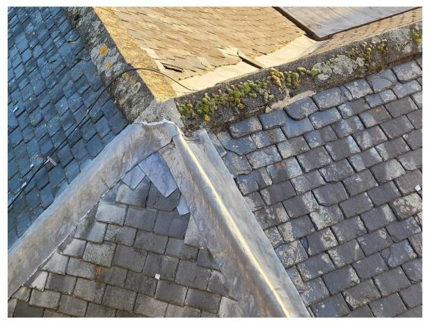
Figure 32. Showing the lead detail at the ridge of the front section.
