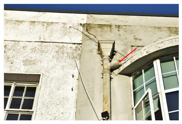
Figure 15. Showing the hopper/downpipe detail at the southeast bay. The bay window outlet is leaking.
