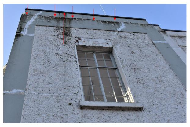
Figure 12. Showing the horizontal step and note the staining due to the flashing spilling onto the plaster. The wall is damp inside this location.
