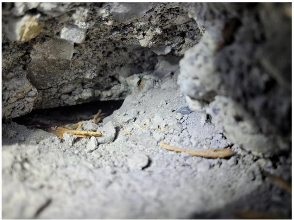
Figure 21. Showing where PJ Barrett widened the crack in a small area showed the crack is full width.
