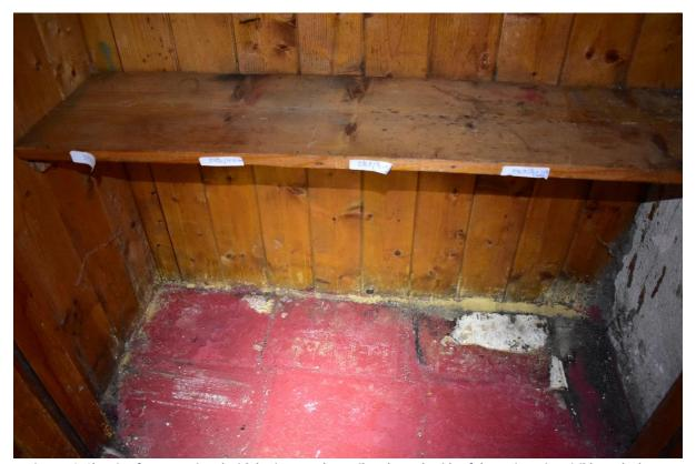
Figure 18. Showing frass associated with boring wood weevil at the underside of the main stairs, visible at the lower ground floor area.
