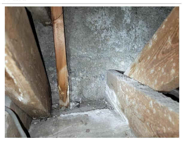
Figure 8. Showing the parapet ceiling joist/wallplate detail.
