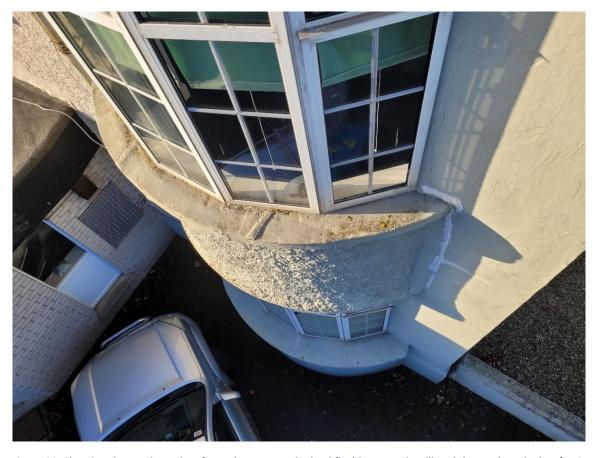
Figure 38. Showing the southeast bay from above. Note the lead flashing over the sill and the crack at the bay/main building junction.
