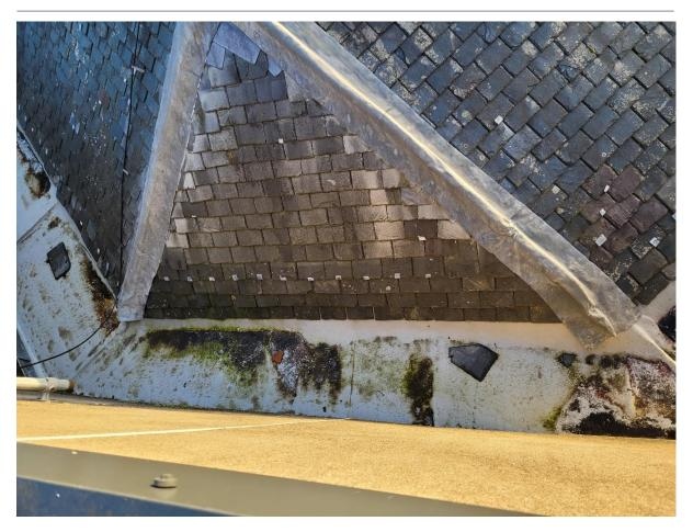
Figure 33. Showing the poor lead detail at the hip ridge
