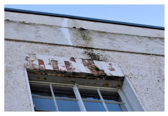
Figure 14. Showing the staining due to water running off the joint of the coping and decaying the brick lintel.
