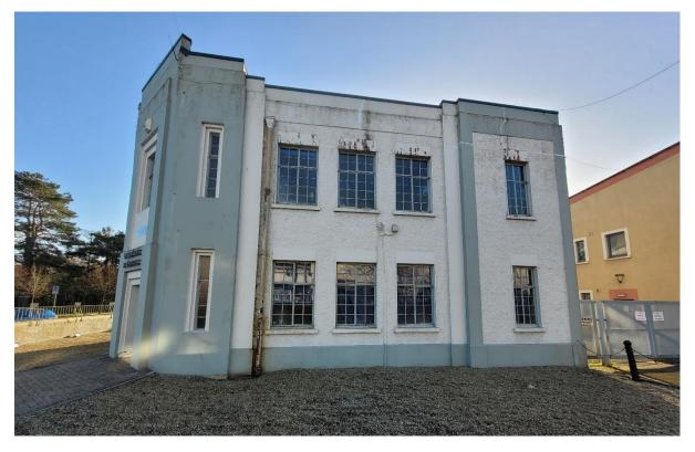
Figure 16. Showing the leaking downpipe at the base. The wall is damp directly adjacent internally.
