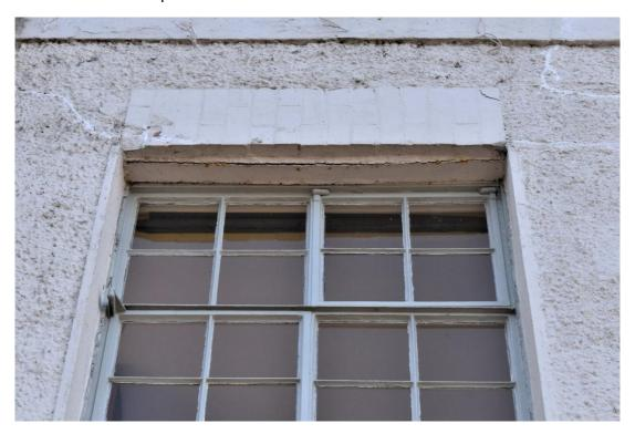
Figure 13. Showing the catnic/lintel at the first-floor level. Note that the lintel is sagging at the centre, and this area corresponds with the internal opening up works.
