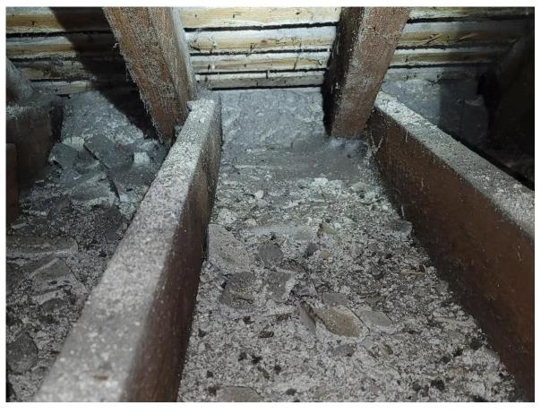
Figure 9. The detail at the rear shows the rafter and ceiling joist penetrating into the concrete.
