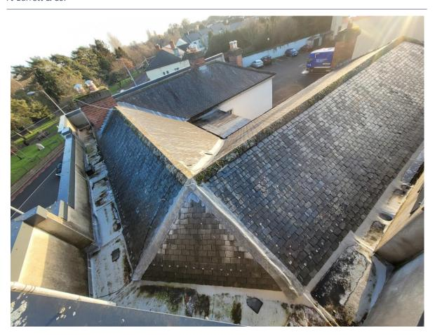
Figure 31. Showing the front section of roof looking south. Note the lead tingles at the fourth row of slates.
