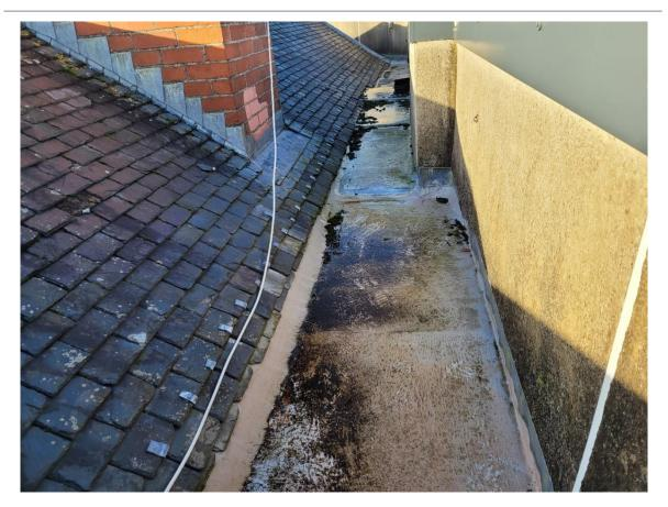
Figure 37. Showing the fibreglass parapet gutter.
