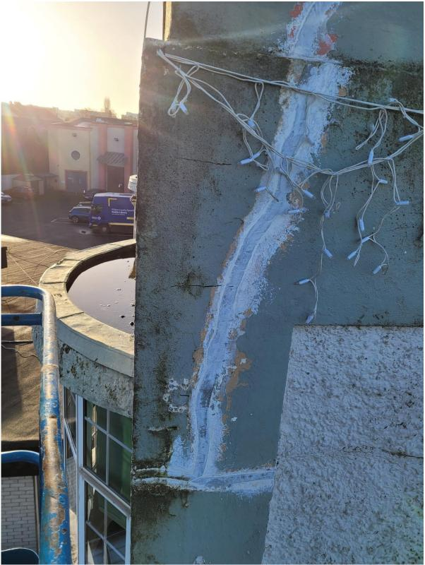
Figure 23. Showing Area 3 looking west. We have marked the holes on site. Note the white filler applied recently.
