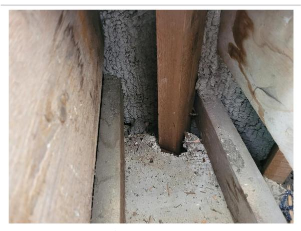
Figure 4. Showing the joist/stud detail forming the external skin of the bay window.
