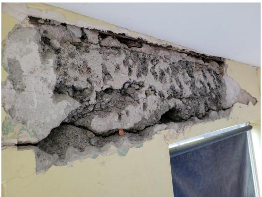
Figure 19. Showing the crack opened up as per Aecom Detail 04.
