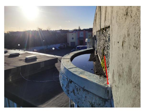
Figure 5. Showing the water lodging at the southeast bay. The roof appears to be leaning out, and there is a crack filled in at the main wall junction.
