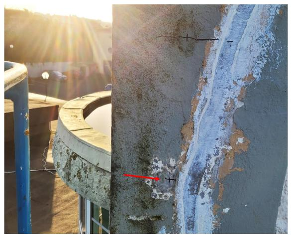
Figure 24. Showing a close-up view of Area 3 looking west. We have exposed the grout at the lower hole.
