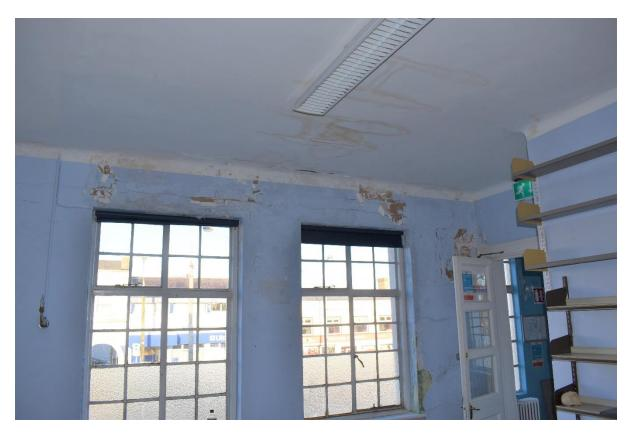
Figure 6. Showing the northwest facing wall in the first floor Book Repository. Note the gypsum plaster is in poor condition.
