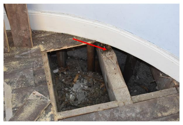
Figure 3. Showing the southeast bay window. Note the decayed 225X75 timber.
