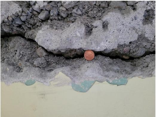
Figure 20. Showing the width of the crack (8-10mm) corresponding with the above image.
